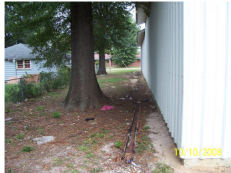
KFC Warehouse, Eastern and School St -evidence of homeless and prostitution
