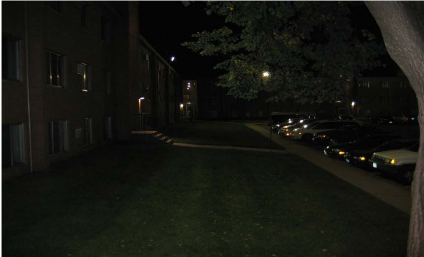
Main entry side shot before
