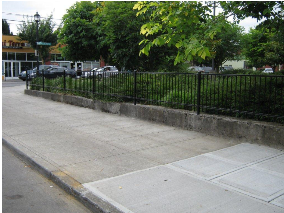
FIGURE FIVE – THE WALL AFTER IMPROVEMENTS
